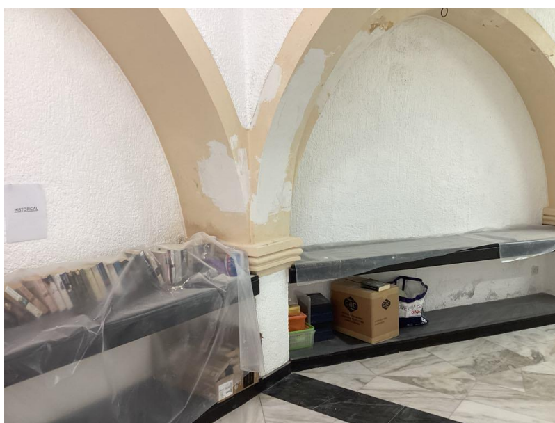
Walls etc being prepped for painting at last
